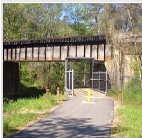
Under Railroad Bridge
